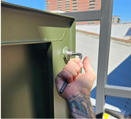
Tighten M10x25 capscrews by hand, but not too tight to allow for movement of the door hinge.
