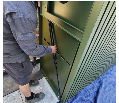
After attaching the door, the door struts can be attached (note orientation).
