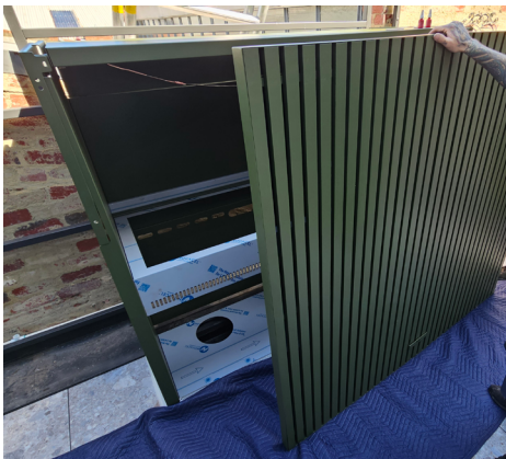
Lay blanket on the ground full length of the Tilt, flush with bottom shelf. This will stop the bottom of the door getting scratched, and act as a buffer to make it easier to mount.
