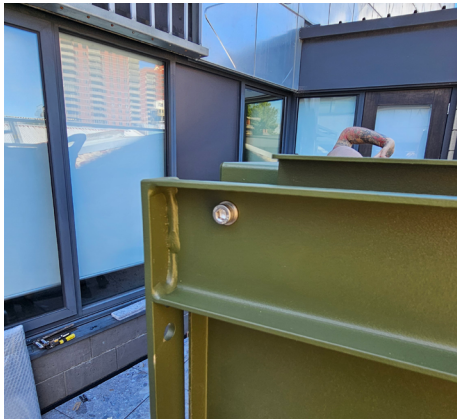
M6 capscrew and washer on outside of hinge.
