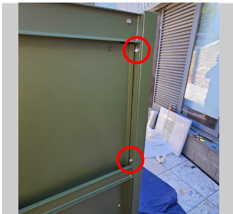
Use M8 button head screws with loctite to attach door to the hinge each side (note locations). You will have access to 2 holes per side, door may need to be moved slightly to find holes. Do screws up tight, being careful of over tightening.
