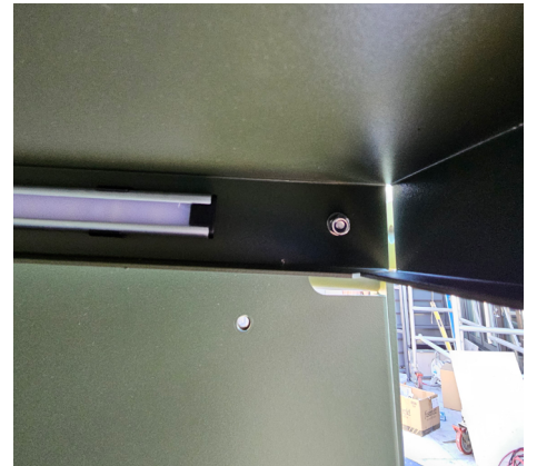
Nylock nut and washer on inside of roof panel.
