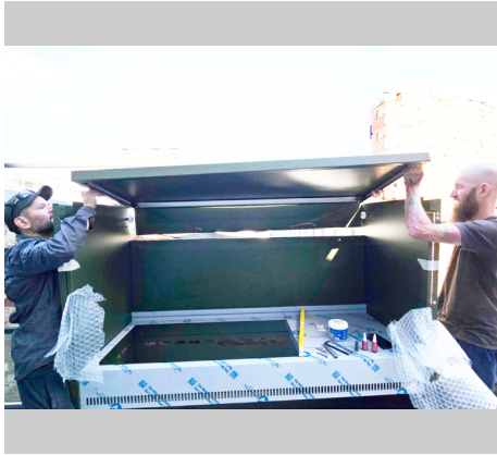
Lift roof panel over Tilt and sit on side panel wheels. Support roof panel in the middle while panel is being fixed to the hinge brackets.
