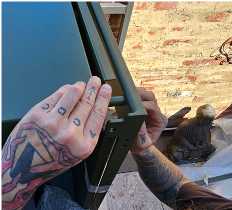
To fix, use spacers with M6 capscrew and a nylock nut. Use washers under head of capscrew and under nylock nut only. Tighten enough so that panel pivots freely.
